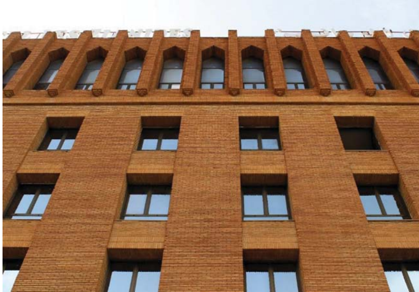
Figure 11 : Detail of the main façade. This image shows the Nedroma red brick cladding, which provides the building's "fortified" texture and thermal mass, layered over the modern reinforced concrete structure. (Author's photo, August 2025)
