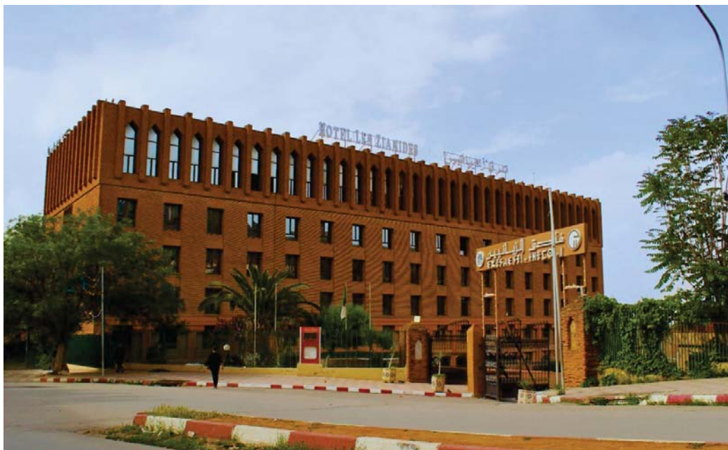
Figure 10 : The principal façade (Author's photo, 2025). This view confirms the material and compositional logic shown in the elevation (Fig 9): (1) the recessed concrete base, (2) the main body in Nedroma red brick, and (3) the arched crowning elements.
