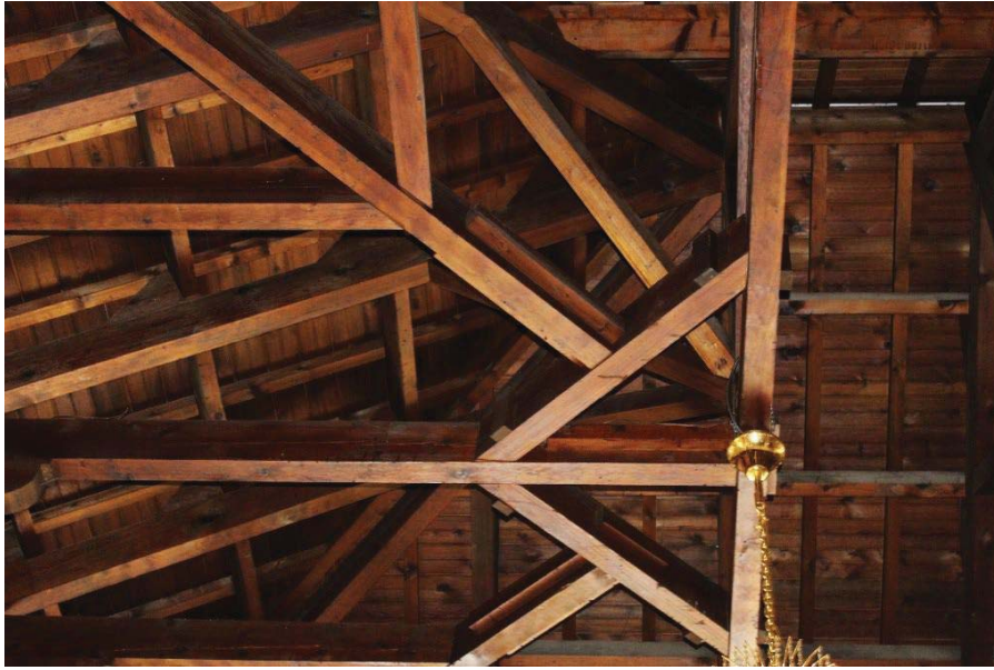
Figure 18 : Modern Reinterpretation: The hotel restaurant's roof structure. Pouillon translates the traditional wooden carpentry (cf. Fig 19) into a modern, double-nave structure. (Author's photo, August 2025)
