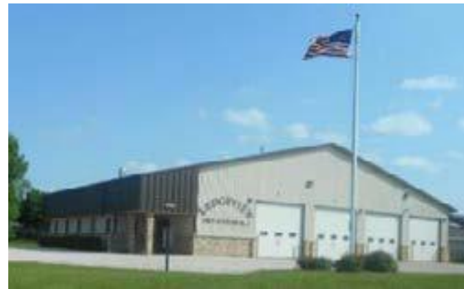
Figure 6.7: Ledgeview Fire Station #2
