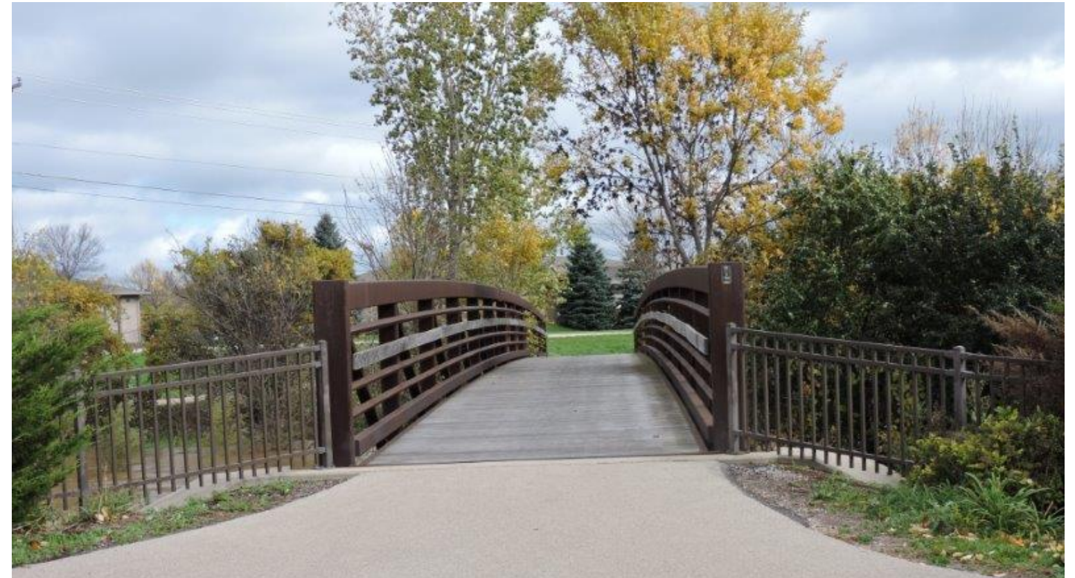
Figure 3.15: Ledgeview Road Bridge over East River
