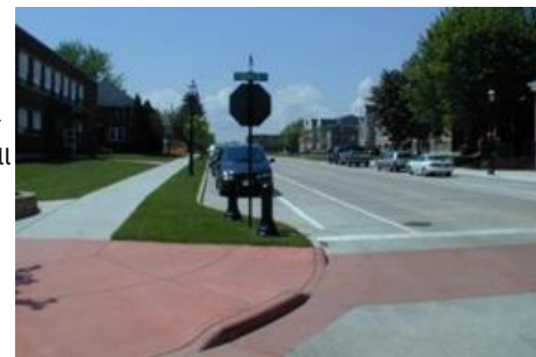
Figure 3.24: Curb extensions provide traffic calming and shorten the distance pedestrian have to cross the street. Grant Street in De Pere shown here. Image: Brown County.
