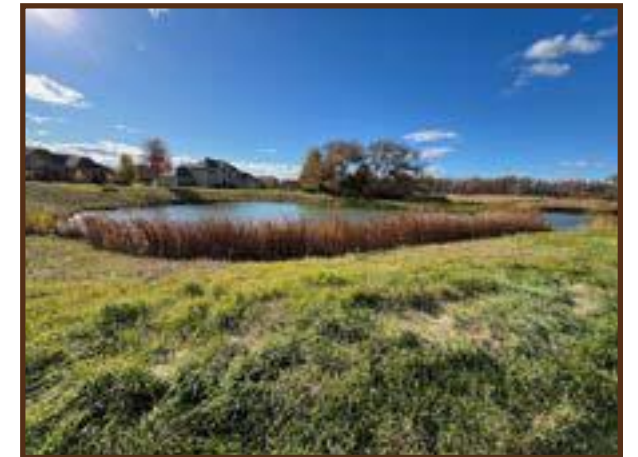
Figure 6.1: Town Stormwater Pond.
