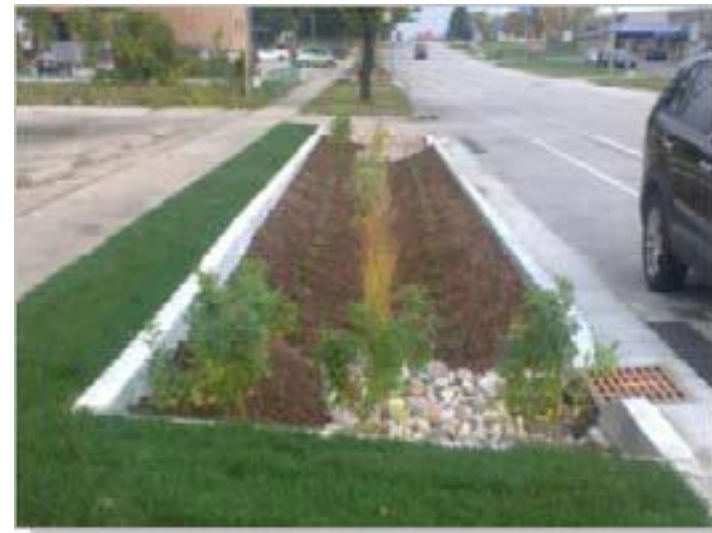
Figure 6.2: Bioswale Example. Source: Source - City of Milwaukee Green Streets Stormwater Management Plan
