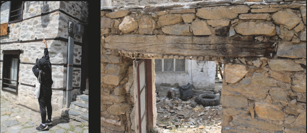
Figure 66-68: (Above) Construction details from a houses along Charshiyska street showing external load-bearing walls (50-60cm wide) construction using stone layering with horizontal timber elements for masonry levelling (typically every 60cm height). (Bellow) Axonometric view from the 3D model of Kalajdzhieva house, (Right) exposing internal arrangements and construction elements (Authors own, 2025)
