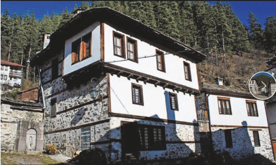
Figure 46: Archival photo of house 6 along Charshiyska street showing the facade of the houses before the restoration effort .(Kyoseva, 2017)
