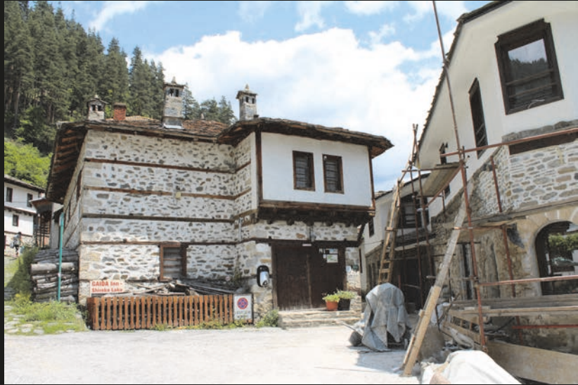
Figure 37-38: (Above) Current photo of houses 1-3 along Charshiyska street (Bellow) 3D render of the current state of the houses .(Authors own, 2025)
