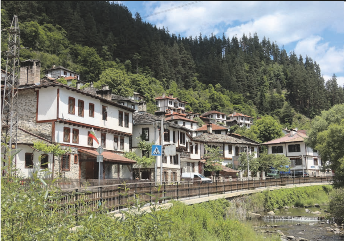
Figure 19: View walking along Petko Voivoda street (Authors own, 2025)
