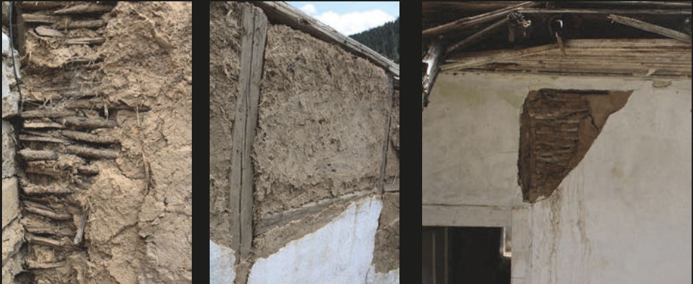
Figure 69-71: (Above) Construction details from a house in ruins along Charshiyska street showing internal partition wall construction using wattle-and-daub walls (clay with straw mixture onto wooden lattice). (Bellow) Axonometric view from the 3D model of Kalajdzhieva house, (Right) exposing internal arrangements and construction elements (Authors own, 2025)
