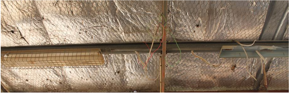
Figure 70-76: Structure and facilities of community hall
