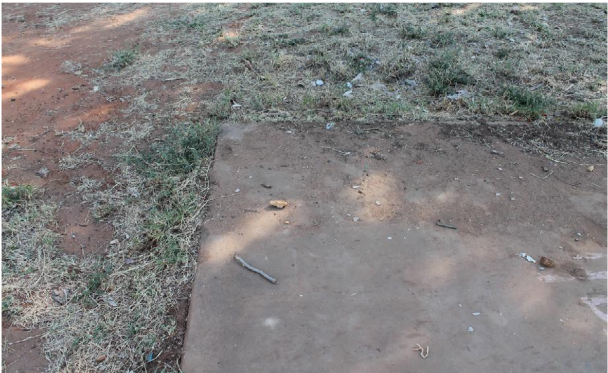
Figure 47: Edge of court slab
