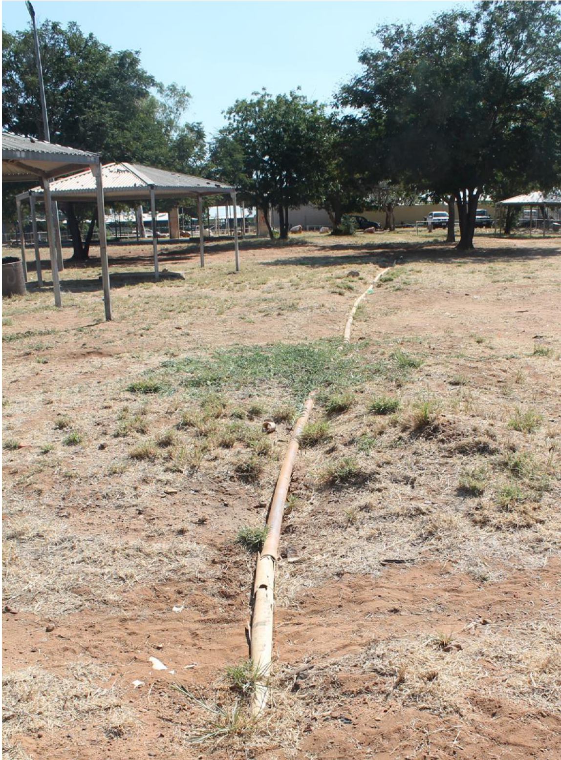
Figure 78: Exposed water pipes located next to courts
