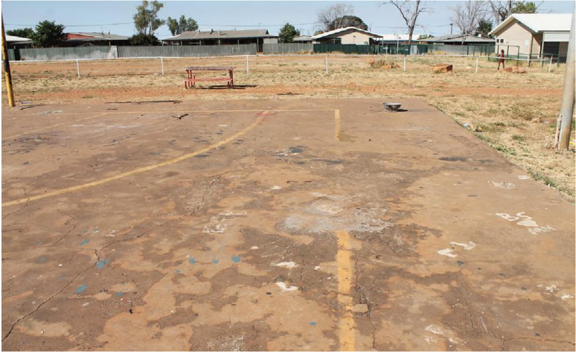
Figure 44: Condition of concrete slab
