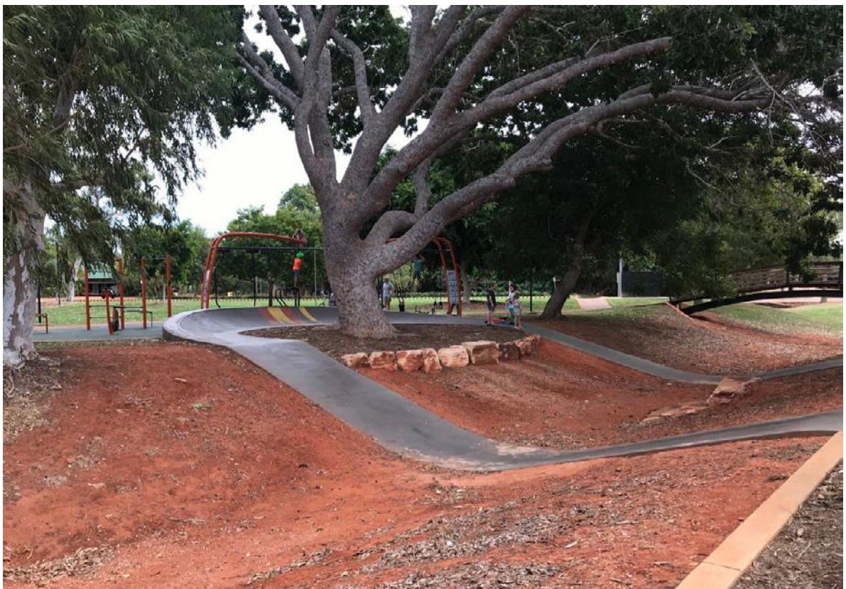
Figure 92-93: Track built along the slopes of existing terrain
