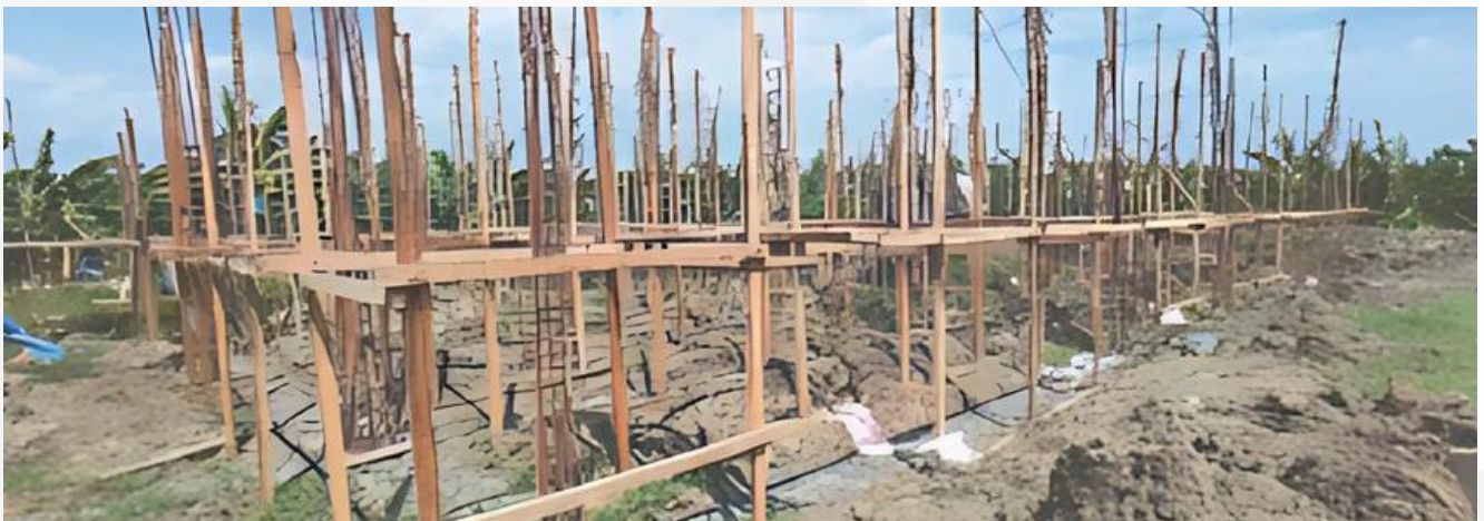
On-going construction of building in DNSC Sto. Tomas Campus.
