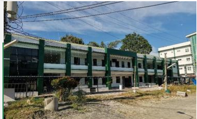
2-Storey Academic Building
