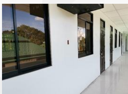
Doors and Windows
