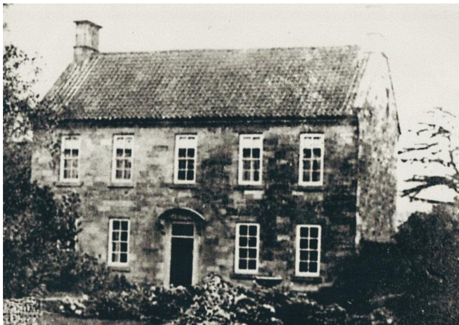
Bridgeholme Green Mansion, built c.1743.
