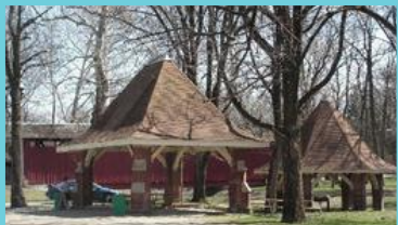
Highland Wellhouse Shelters
