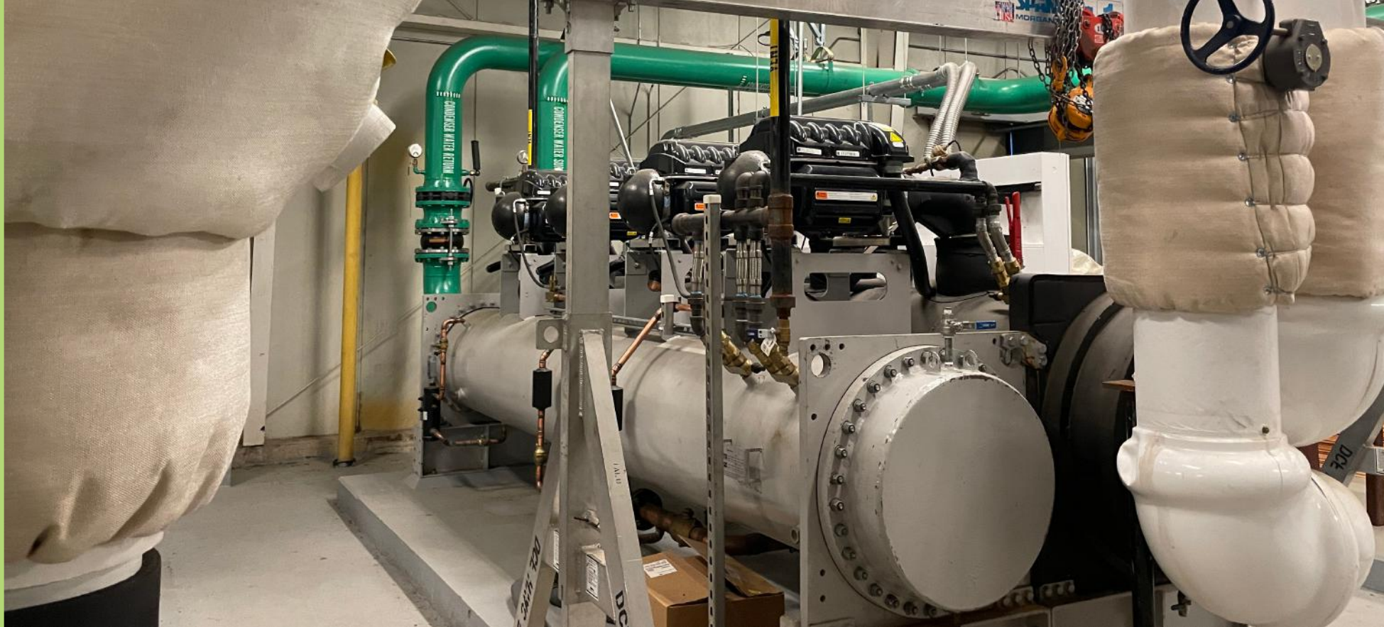
Image 3.5: Chiller for West Campus chilled water loop, located in the Powerhouse.
