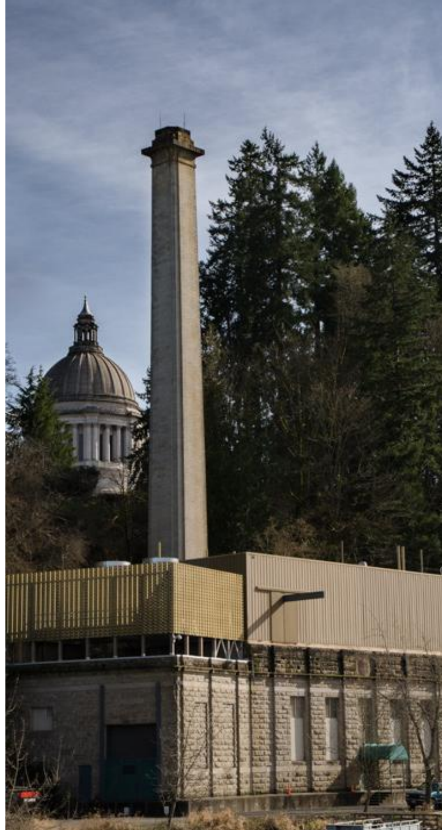
Image 3.2 (above): Powerhouse Building.
