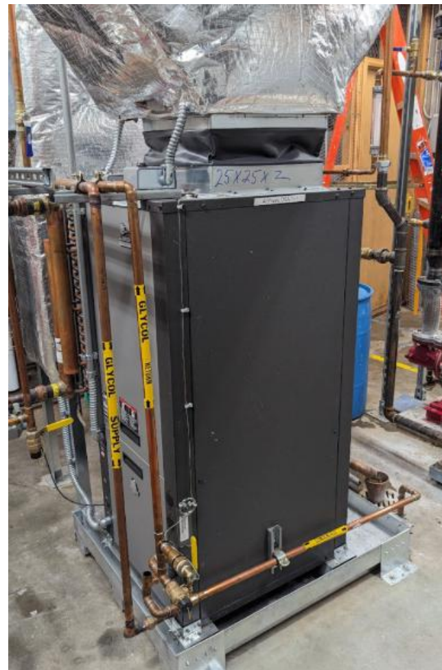
Image 8.7 (left): Heat pump fan coil unit in Archives Building.
