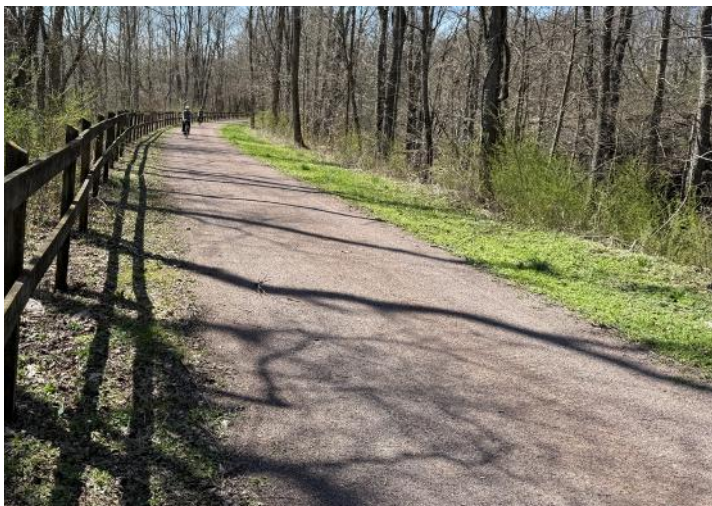
Above: Example of regular trail surface grooming: the crushed gravel surface is free of ruts and grass growth.
