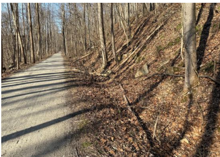
Above: Accumulated leaf litter and fallen branches can reduce a swale's depth and ultimately its efficacy.
