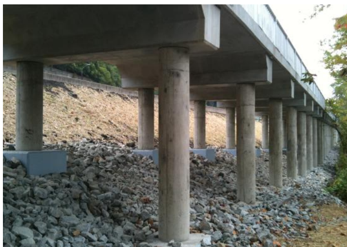
Above: A concrete boardwalk constructed for the Three Rivers Heritage Trail in Pittsburgh, PA.
