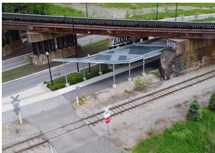
Above: This structure was constructed under an active railroad bridge to catch any potential debris falling onto trail users from rail cars.
