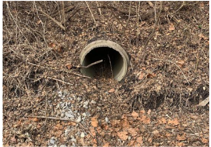
Above: Ensuring that the outlets of pipes and culverts are not blocked by debris is an ongoing maintenance challenge.
