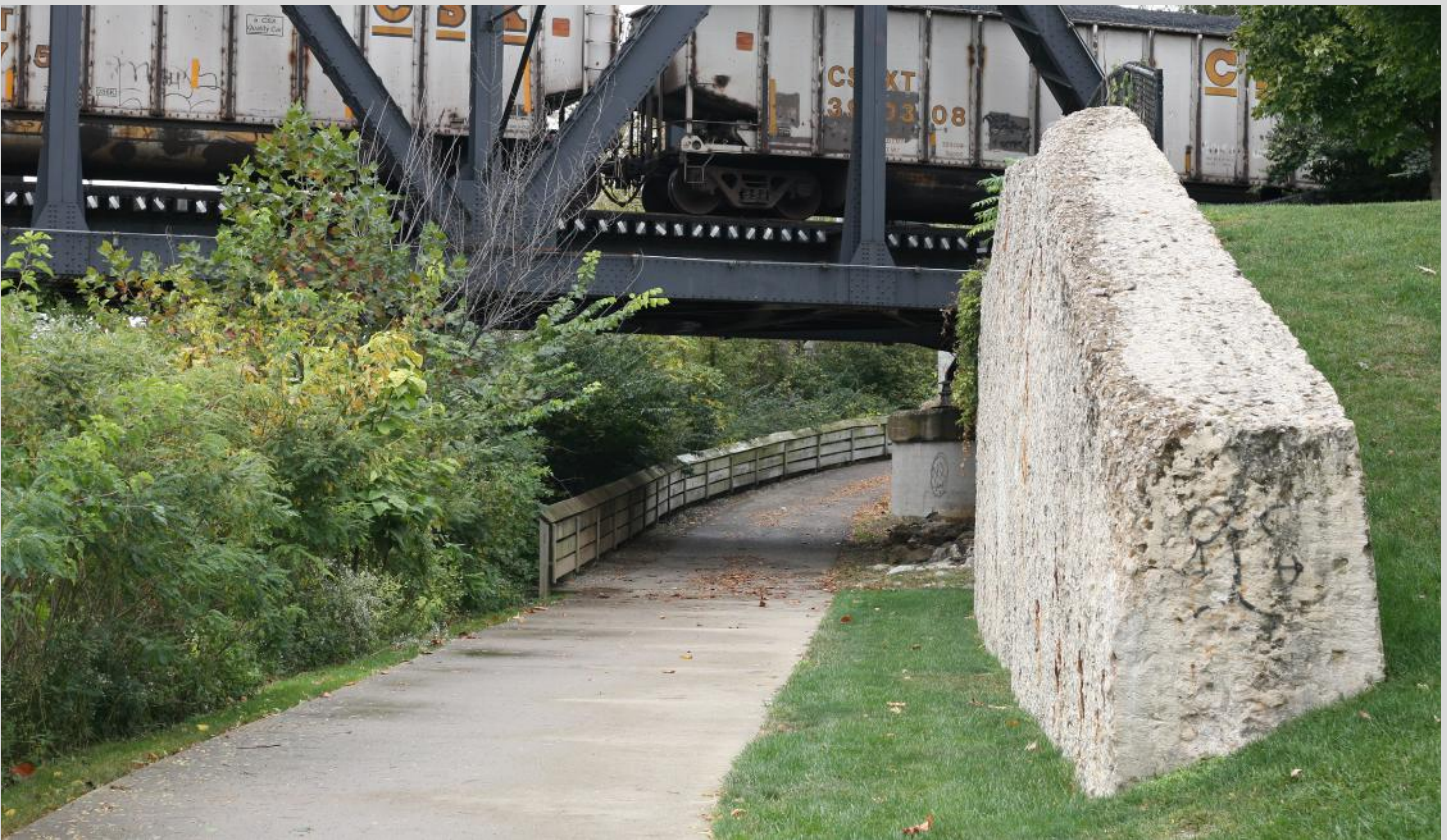
Top left: The Canoe Creek State Park to Lower Trail connector underpass. Blair County, PA. (Photo credit: Rails to Trails of Central PA.)
