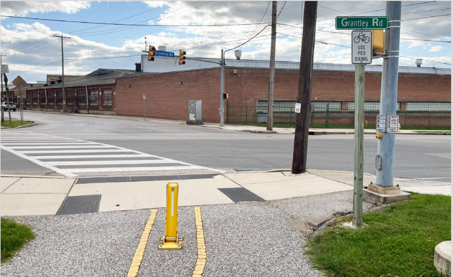
Top left: This trail crossing for the Capital Area Greenbelt in Harrisburg, PA includes permeable pavers.
