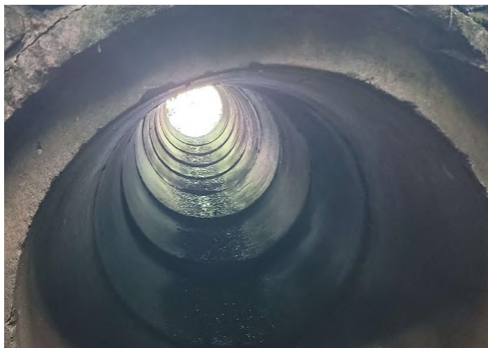
Above: A look inside a concrete pipe.
