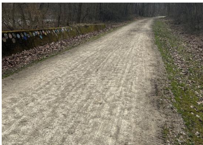
Above: This crushed gravel trail is deceptively bumpy, and debris like what's in the center of the trail gets trapped easily in bicycle spokes.
