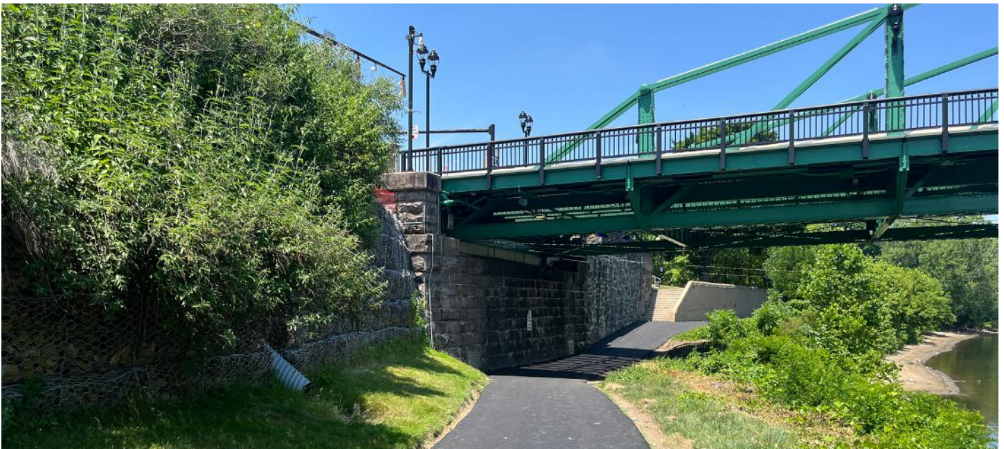
Above: An underpass along the Two Rivers Trailway in Easton, PA, just across the Delaware River from New Jersey.
