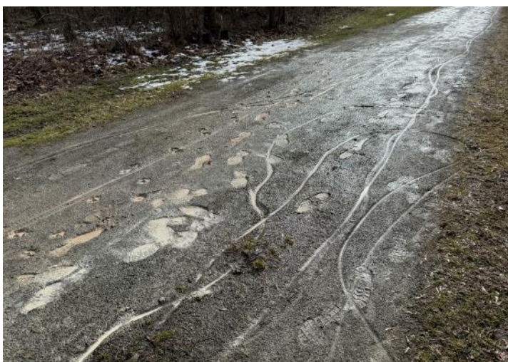
Above: Crushed gravel trails, particularly in shady locations, are prone to rain and snowmelt saturation that causes a muddy surface.
