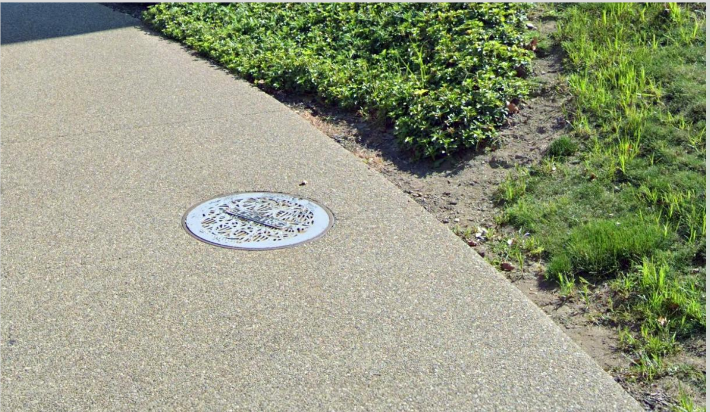
Top left: A circular iron grate with fallen leaves swept away to encourage water to properly flow into the inlet.
