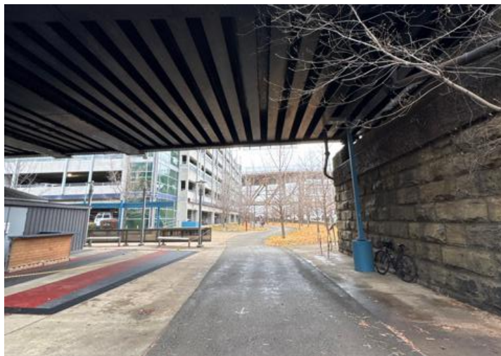
Above: This railroad underpass on the Three Rivers Heritage Trail in Pittsburgh, PA is served by a lighting fixture for better nighttime safety.
