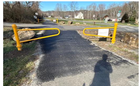
Below: An asphalt fog seal at a trail crossing for the Great Allegheny Passage in Dunbar Township, Fayette County, PA.
