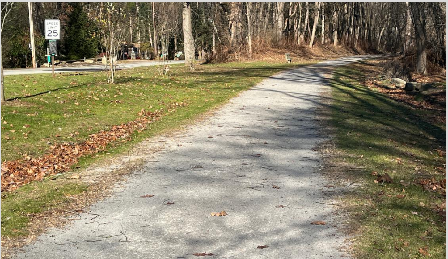
Top left: Detail of crushed limestone. (Photo credit: Sutherland Landscape Center, Chico, CA.)
