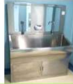
Operating Room Sink
