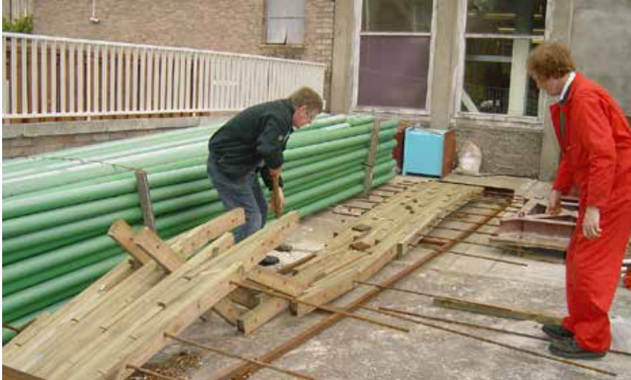
- Dismantling a Stress Laminated Bridge
