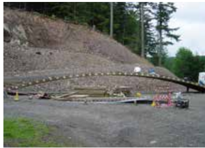
- 20m span test bridge at Glentress during construction
