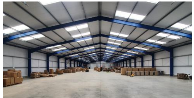
Above: A new 32,000sq ft extension is built in 2020 to house all aspects of production under one roof
