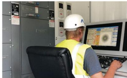
MTBM Operator at Control Console
