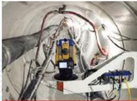
Pipe Station center mounted
