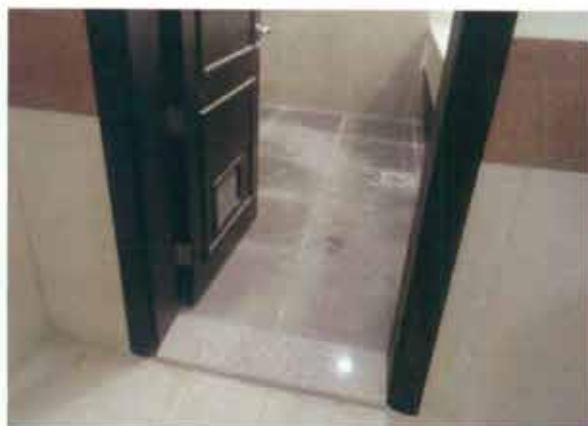
Typical door threshold step
