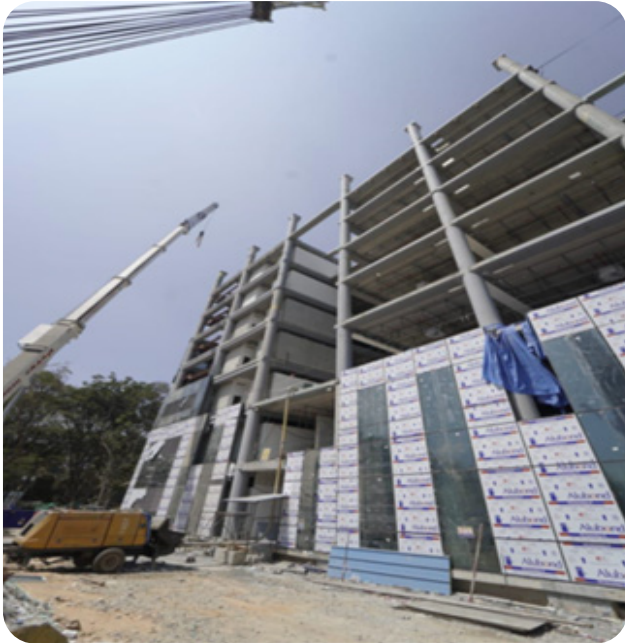
Day 29 & 30, March 1 and 2, Unitized Structural System for the second floor are installed.
