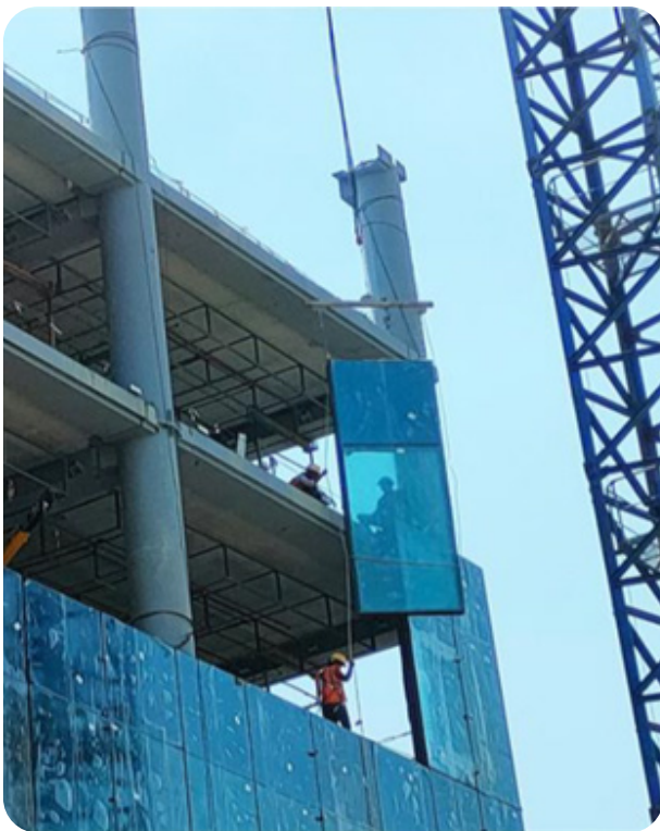
Day 33, March 5, Façade Panels for fifth and sixth floor are installed
