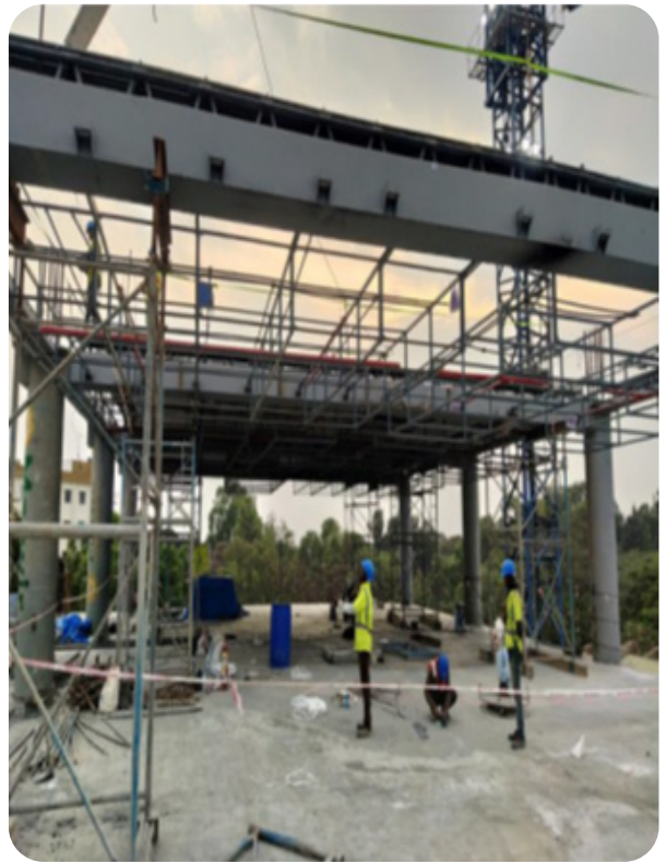
Day 36, March 8, Terrace floor slabs and beams erected.
