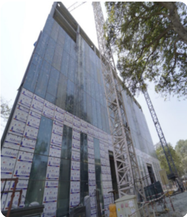
Day 37 & 38, March 9 & 10, Façade Panels fixed in the sixth floor
