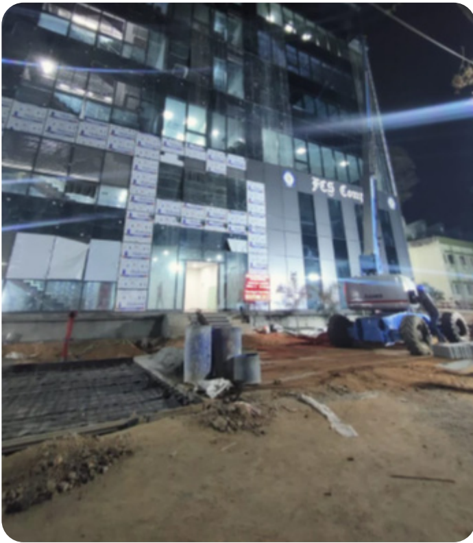
Day 41 & 42, March 13 & 14, Road and external electricification , water supply and sewage works completed
