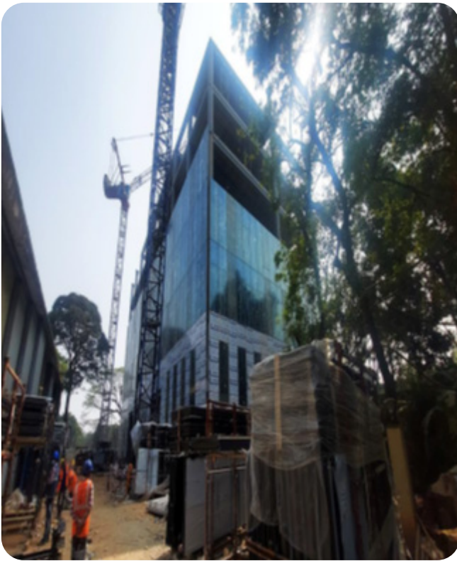
Day 35, March 7, Façade panels fixed in the fourth and fifth floor.
