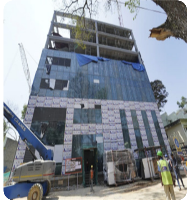
Day 31 & 32, March 3 and 4, Unitized Structural System for the third floor are installed.
