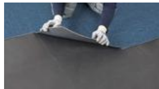
Apply planks or tiles
