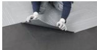
Apply planks or tiles
