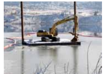
Ready to install the intake and pipeline.
