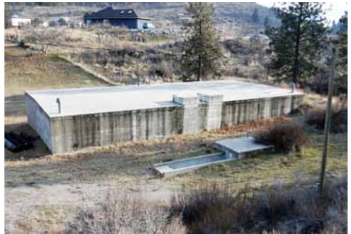
Cypress Reservoir and valve chamber.
