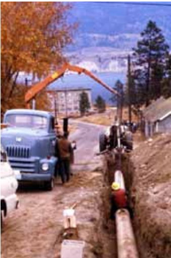
Laying pipe up Lakehill.
