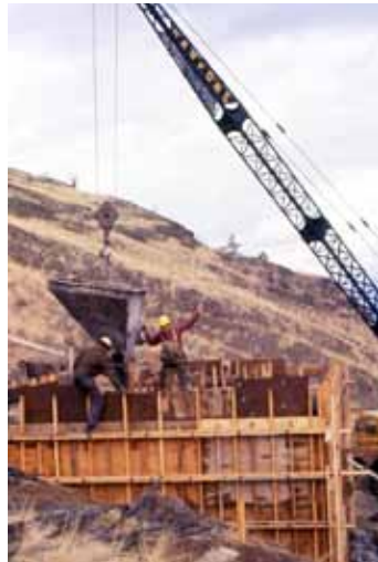
Constructing Greyledge head tank.
