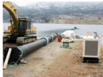
Fabricating the intake and pipeline.
