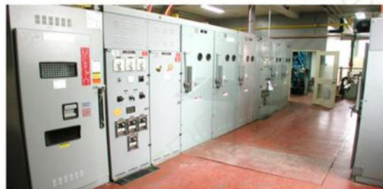
Extinguishing local electrical factory fires
