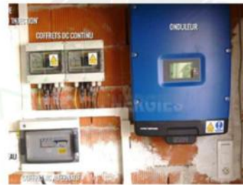
Fire extinguishing for DC / AC box connecting photovoltaic panels
