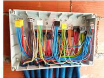
Fire extinguishing for junction box
