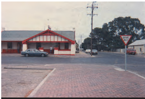
Normanville Hotel before renovations & extensions.
