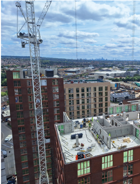
Prefaxis twin walls were used for the stairway cores and lift shafts in this apartment development in London
