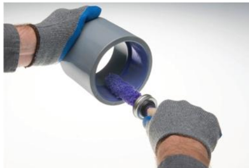
Apply primer to ID of fitting
