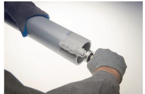
Apply cement to OD of pipe
