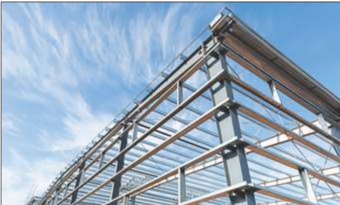
PPG Steelguard 951 coating provides up to four hours of fire protection by expanding from a thin, lightweight film into a thick, insulating foam.
