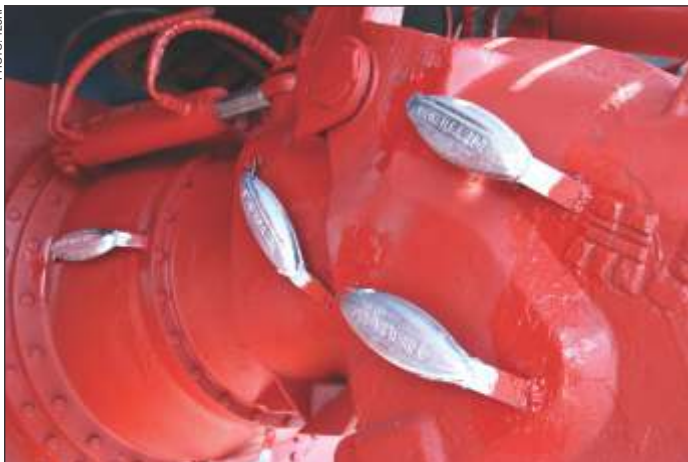
Carbon black is a conductive fillers or additives used in cathodic protection systems.
