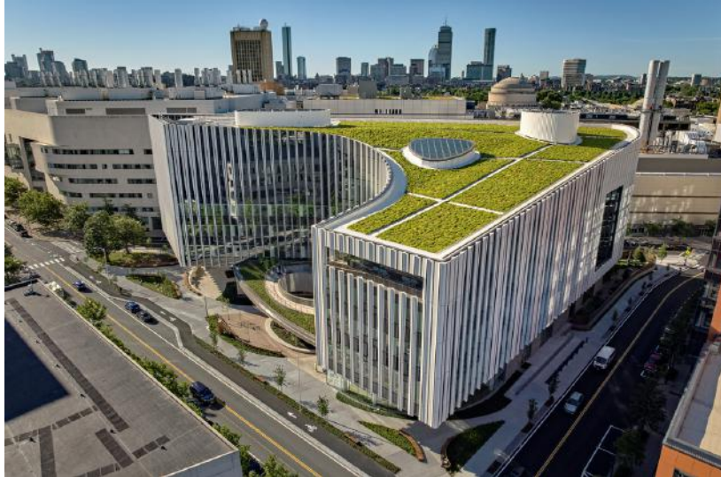
Ragon Institute of Mass General Brigham, MIT, and Harvard Cambridge, MA | 2024 Payette | Consigli Construction LEED Gold Certified Photo Credits: Robert Benson Photography
