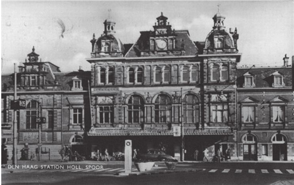
Station Den Haag Hollands Spoor, 1891
