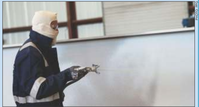
PPG Steelguard 652 cellulosic passive fire protection (PFP) coating delivers up to two hours of fire protection.
