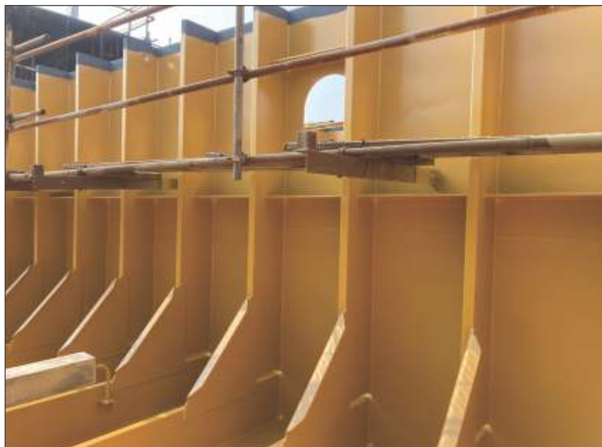
Interior water ballast spaces showing coated internal bulkheads and stiffeners.
