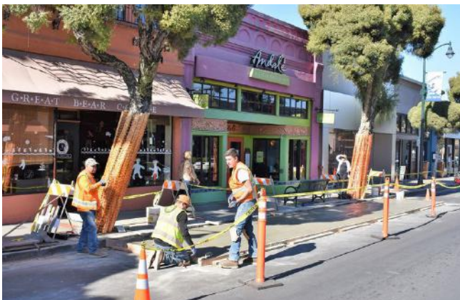
Figure 37: Construction of parklet in Los Gatos, California
