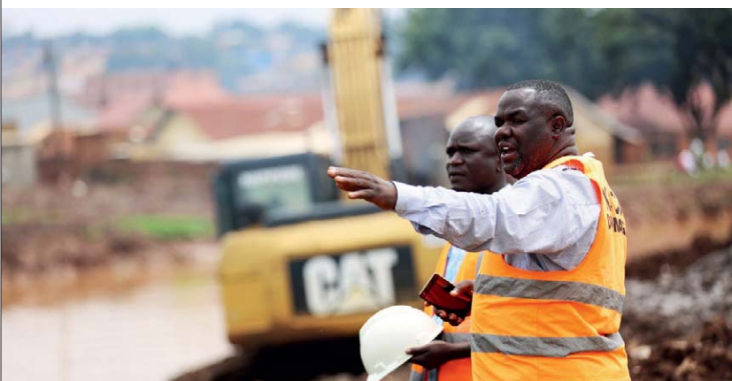
Above: Supervising road construction in Kampala City.
