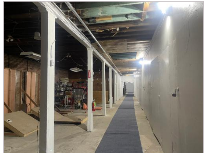
Interior view of the ground floor
