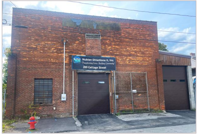
View of the north side of the building from Cottage St
