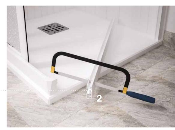
(2) Using a hacksaw with blade pitch not exceeding 2 mm it will be possible to REDUCE the length of the sliding profles.
