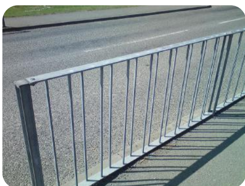
Staggered pedestrian rail without gap
