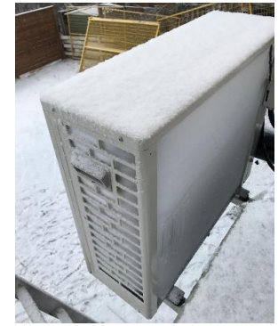
Figure 48: A Sanden CO2 heat pump water heater compressor working outside in 5°F (-15°C) weather. 102
