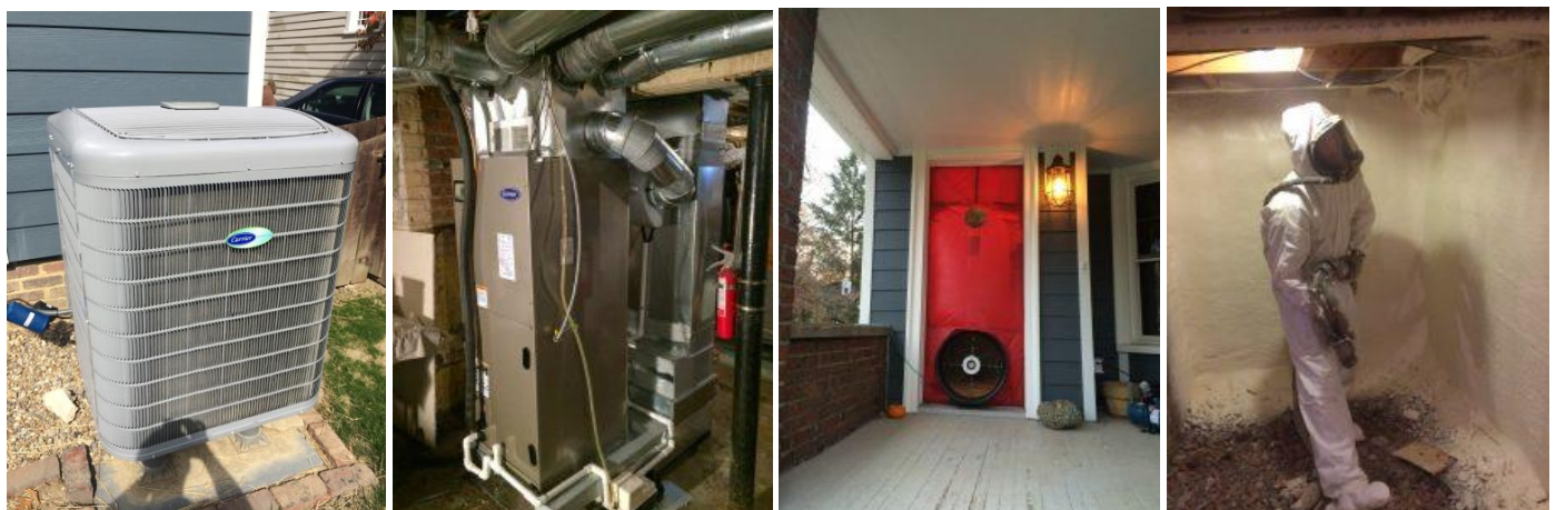
Figure 15: A few images from Energy Smart Ohio’s retrofit project 1918 House of the Future in Cleveland Heights. Left to right: Carrier Greenspeed heat pump, air handler in the basement, blower door test, and insulating the basement.
