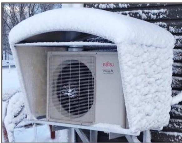
Figure 39: Fujitsu heat pump in the snow. 86
