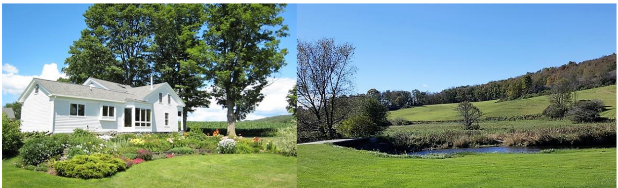
Figure 29: Peter Darby's home that was built in 1830 was retrofitted to be zero emissions and all-electric, including a water source heat pump that uses well water as the heat source, and discharges the water into the adjacent creek. 74
