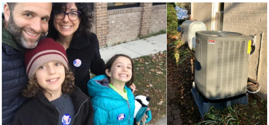
Figure 25: Ben and Sara Shalva replaced their fuel oil furnace with a heat pump for a more comfortable, fossil fuel free house. Multiple neighbors recommended a local installer who had already replaced their fuel oil furnaces with heat pumps, saving utility costs every winter and adding AC to an old house for comfortable summers. 67
