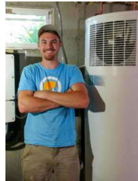
Figure 47: A Steibel Eltron heat pump water heater installed in a basement in the Northeast. 101
