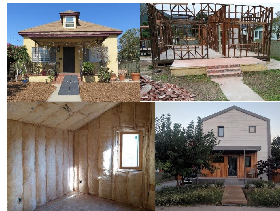
Figure 31: The Perlita Passive House: the original house was stripped to the studs, re-insulated, tested and made into an LA modern masterpiece of efficiency. 76
