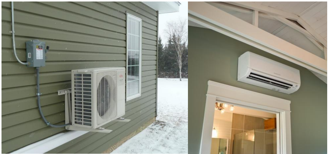
Figure 42: An example of a ductless mini-split heat pump outdoor compressor 95 mounted to stay above the snow and a wall-mounted indoor fan coil 96 .
