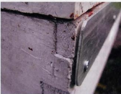
Installing a metal strip with a little added spacing makes a lip to keep the tilted box from falling.
