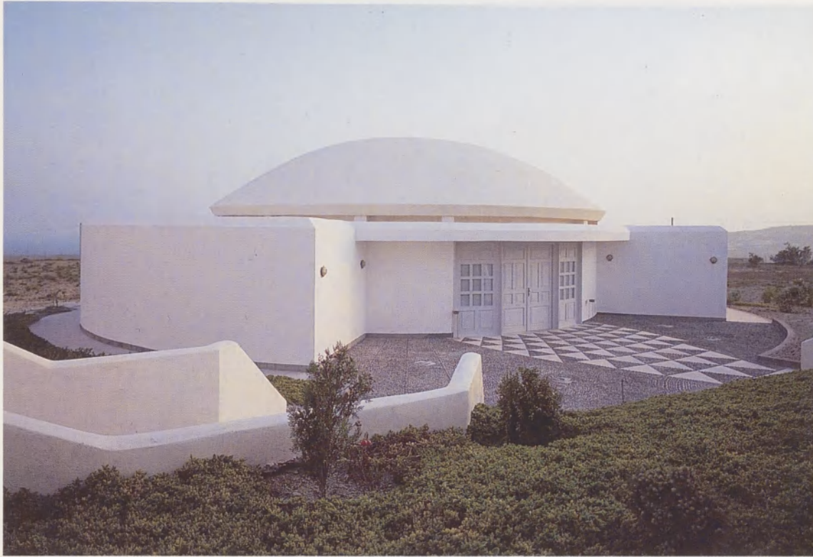
Fig. 83 The 'Tholos' of the Boutari winery. Traditional lines and modern materials.
