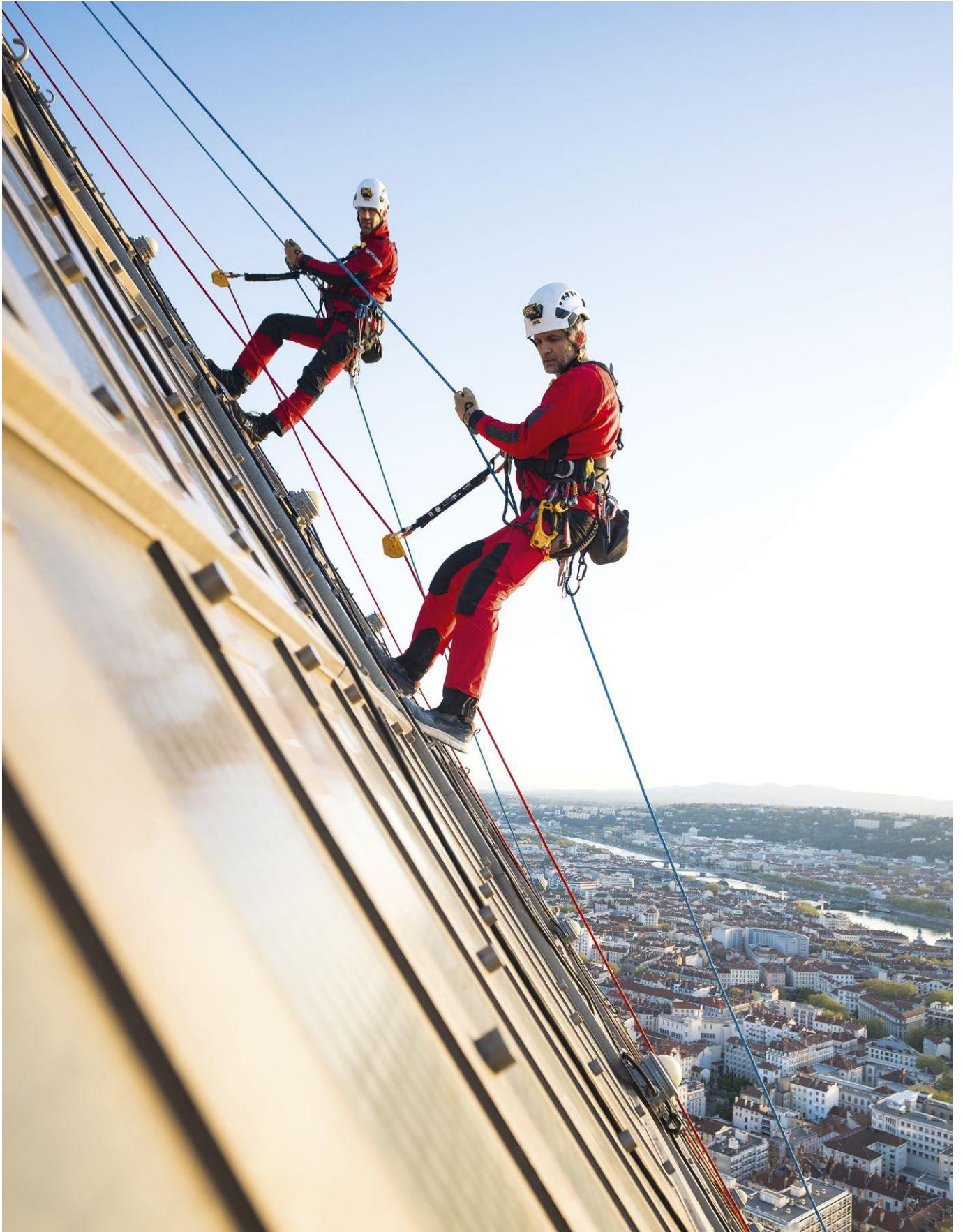
Glass window maintenance, Tour Crayon de la Part-Dieu, Lyon, France © 2024 Petzl Distribution - Vuedici.org - Bleu Ciel Services (BCS) - Tour Crayon de la Part-Dieu
