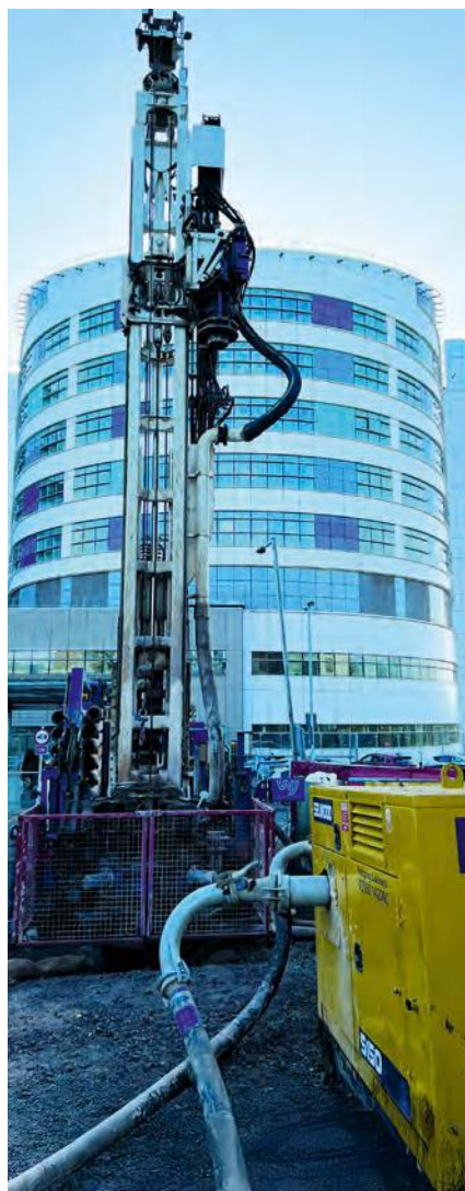
Drilling a borehole ready for an installation
