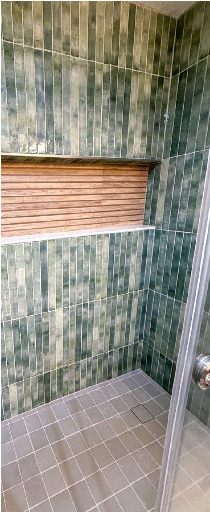
This project included an infinity niche, tiled corner footrest, and tileable shower drain.
