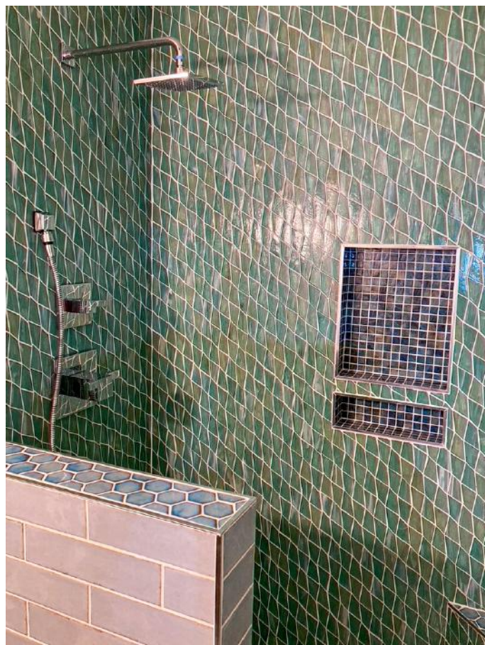
Paper-faced glass mosaic tiles, which Overby’s company set with epoxy grout.
