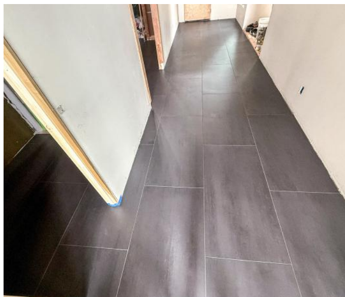
24"x48" 1/2"-thick Mosa tiles were installed in this project.
