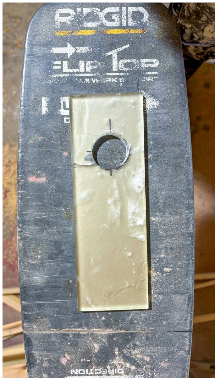
If at all possible, holes for hardware or penetrations should be pre-drilled before installation by the tile or glass fabricator.
