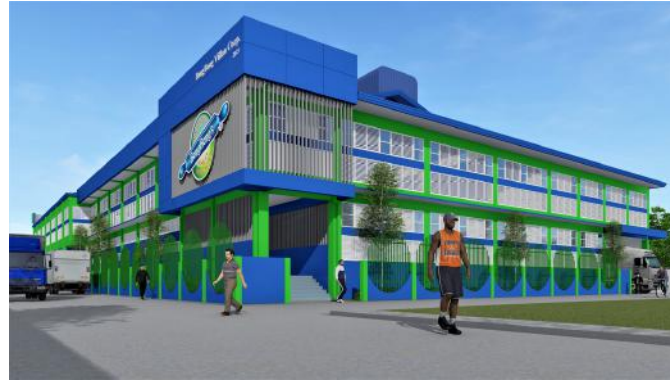
VILLAN BUILDING EXTENSION Brgy. Alijis, Bacolod City
