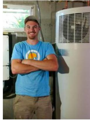
Figure 24: A Steibel Eltron heat pump water heater installed in a basement in the Northeast.<sup>83</sup>
