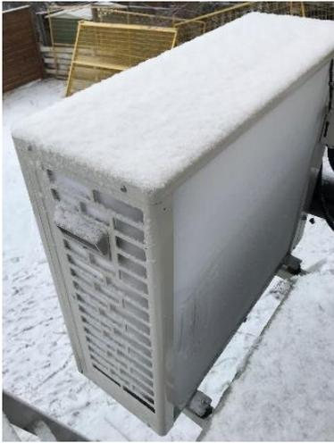
Figure 26: The Eco2 heat pump water heater compressor working outside in 5°F (-15°C) weather.<sup>86</sup>
