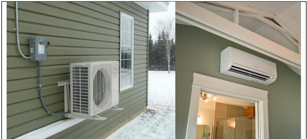
**Figure 30: An example of a ductless mini-split heat pump outdoor compressor<sup>110</sup> mounted to stay above the snow and a wall-mounted indoor fan coil<sup>111</sup>.**
