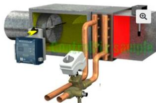
Figure 7: VAV Box with water reheat Coil.
