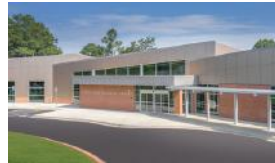
North Cobb Regional Library 3535 Old 41 Highway Kennesaw, GA 30144
