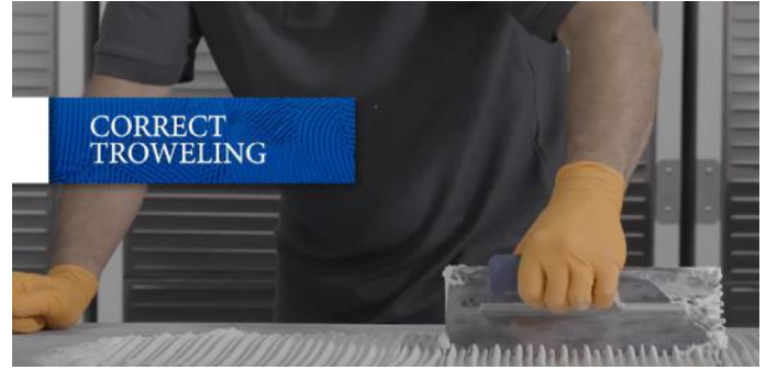
The video illustrates the correct troweling technique – short side to short side.
