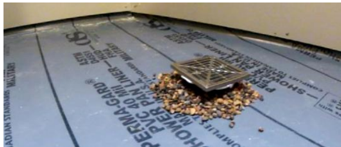
Use of a positive weep protector instead of pea gravel would ensure protection of weep holes.
