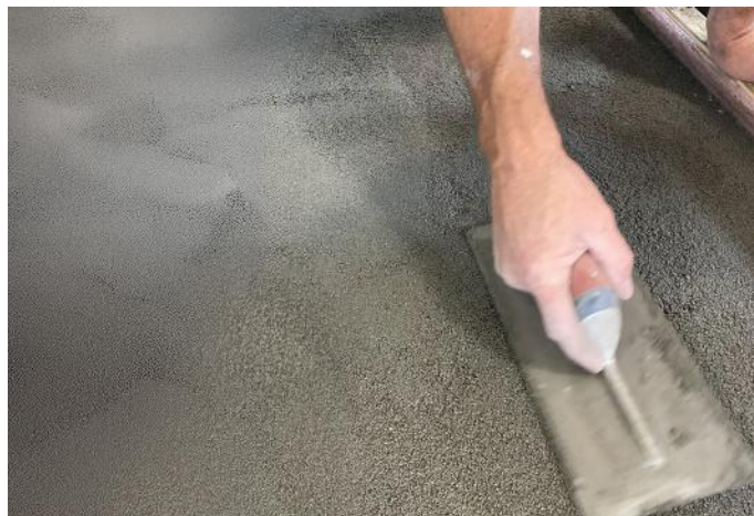
It's important to determine if the original installation is sound before floating over an existing mortar bed.
