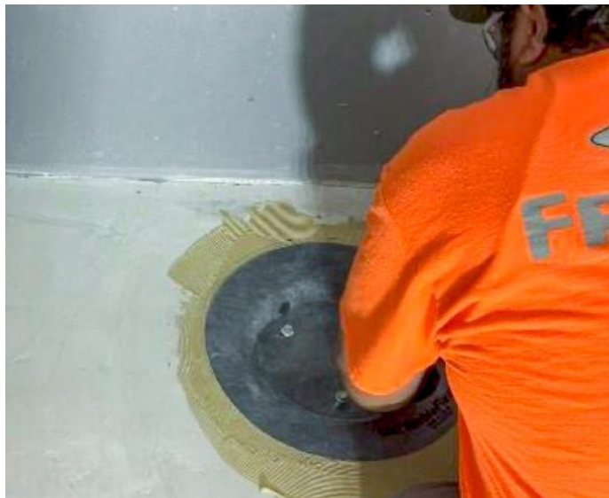
Prefabricated drain flashings are useful when waterproofing ties into this critical drain detail.
