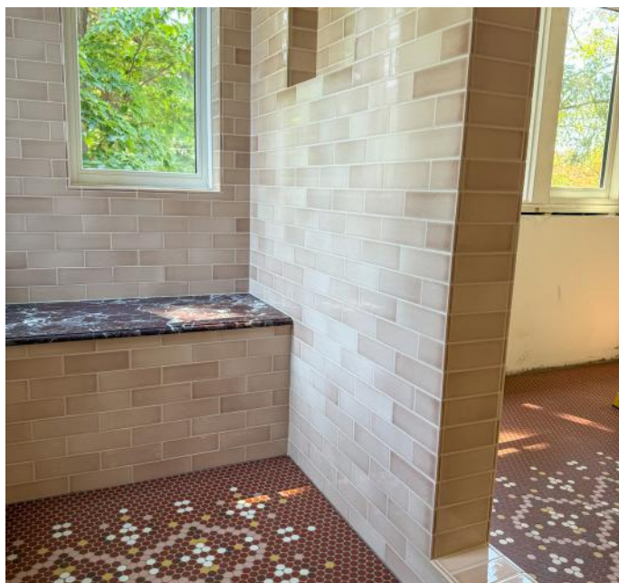
You'd never know from looking at this install how much the floor was out of level when the project began, but Hawthorne Tile made sure the floor was level before beginning the install.
