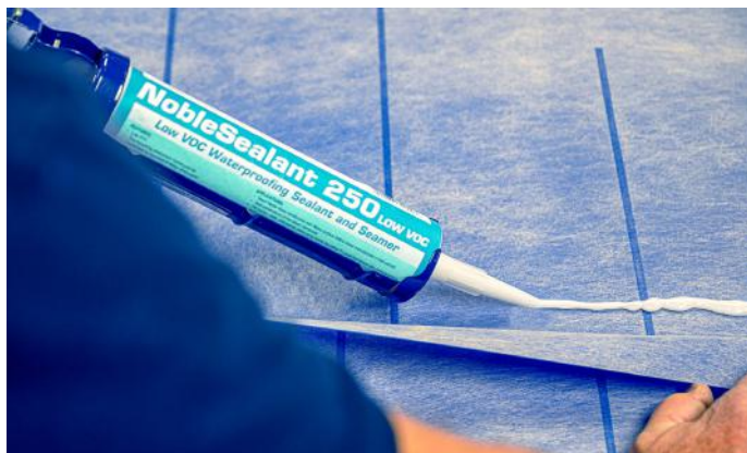
Make sure you use the correct sealant as required by the waterproof membrane manufacturer.
