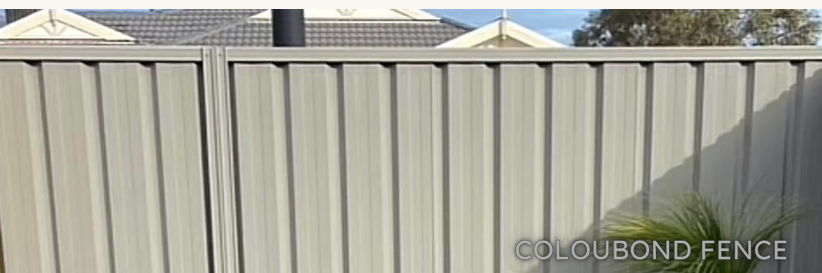
PAILING SIDE OF FENCE
