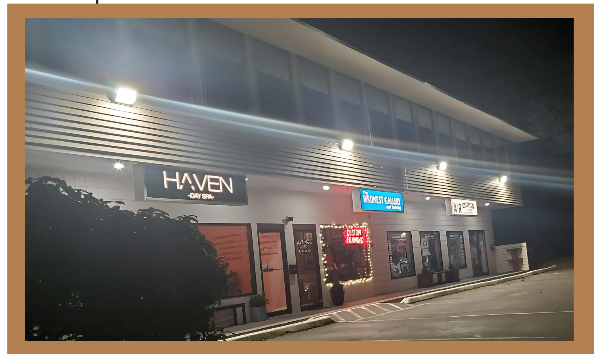
PHOTO OF COMPLETED LIGHTING AT DUSK
