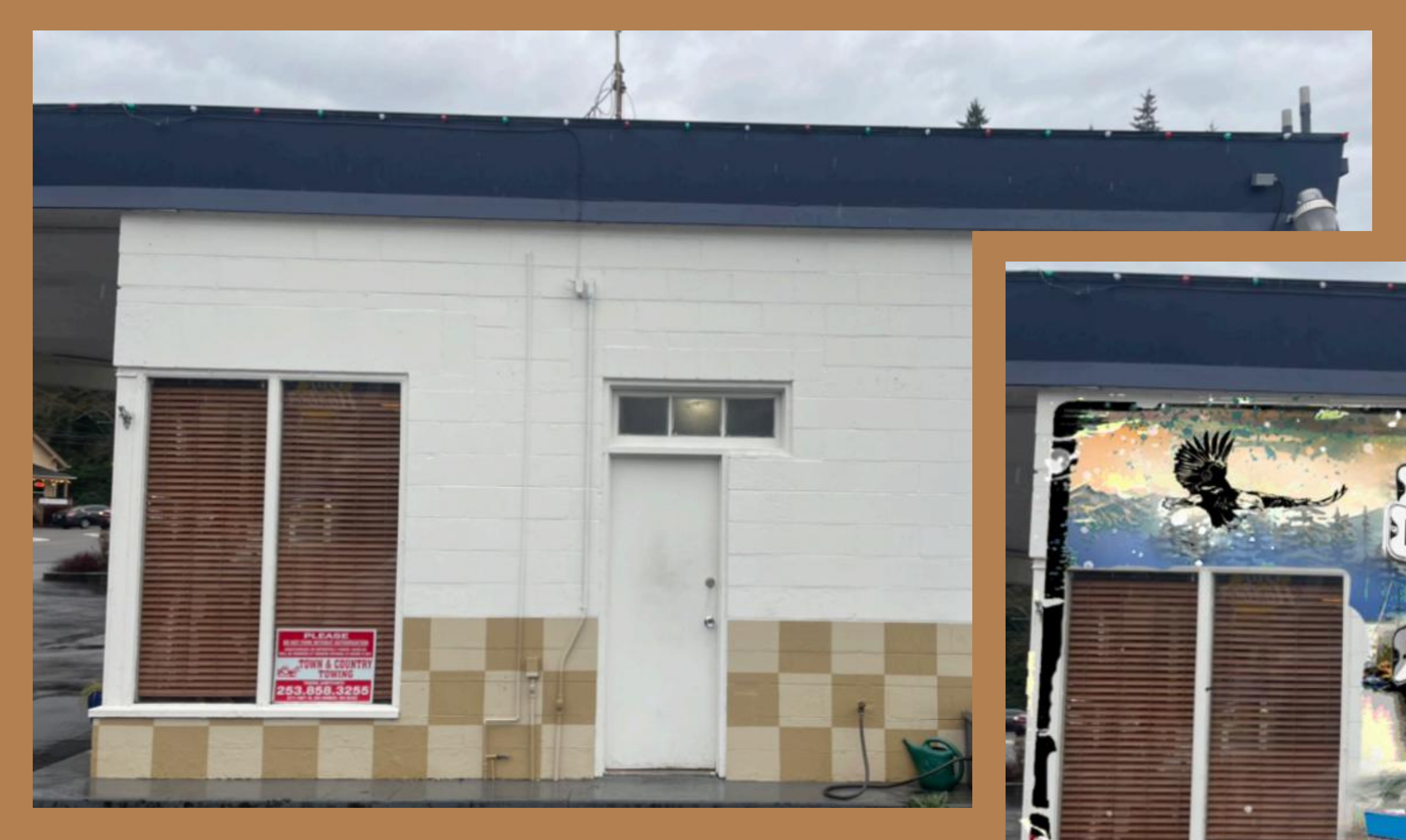
CURRENT VIEW OF PROJECT SITE
