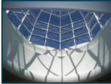
26 roofs to be replaced on an ongoing basis
