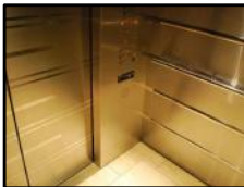
14 elevators to support patron accessibility and productions
