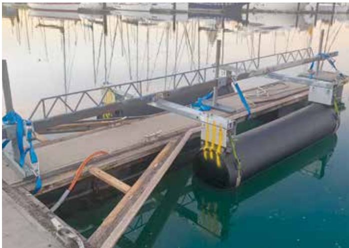
Outrigger in place prior to disconnection
