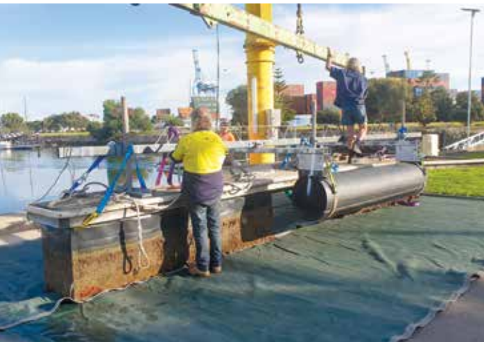
Lifting onto the crane wharf
