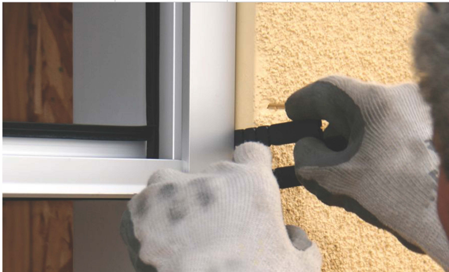
HORSESHOE1/4 Horseshoe Shim Tile Spacers (1/4" Thick)
