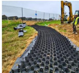
The geocell is a three-dimensional cell that stabilizes soil through confinement. The GEOWEB Soil Stabilization System has an interconnected honeycomb-like network that confines fill vertically and horizontally to prevent lateral shearing and movement for slope stabilization, load support, channel protection and wall reinforcement.
