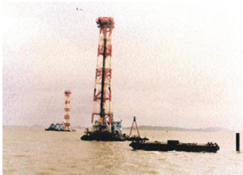
1 PILING MACHINERY INSTALLED FOR JETTY CONSTRUCTION
