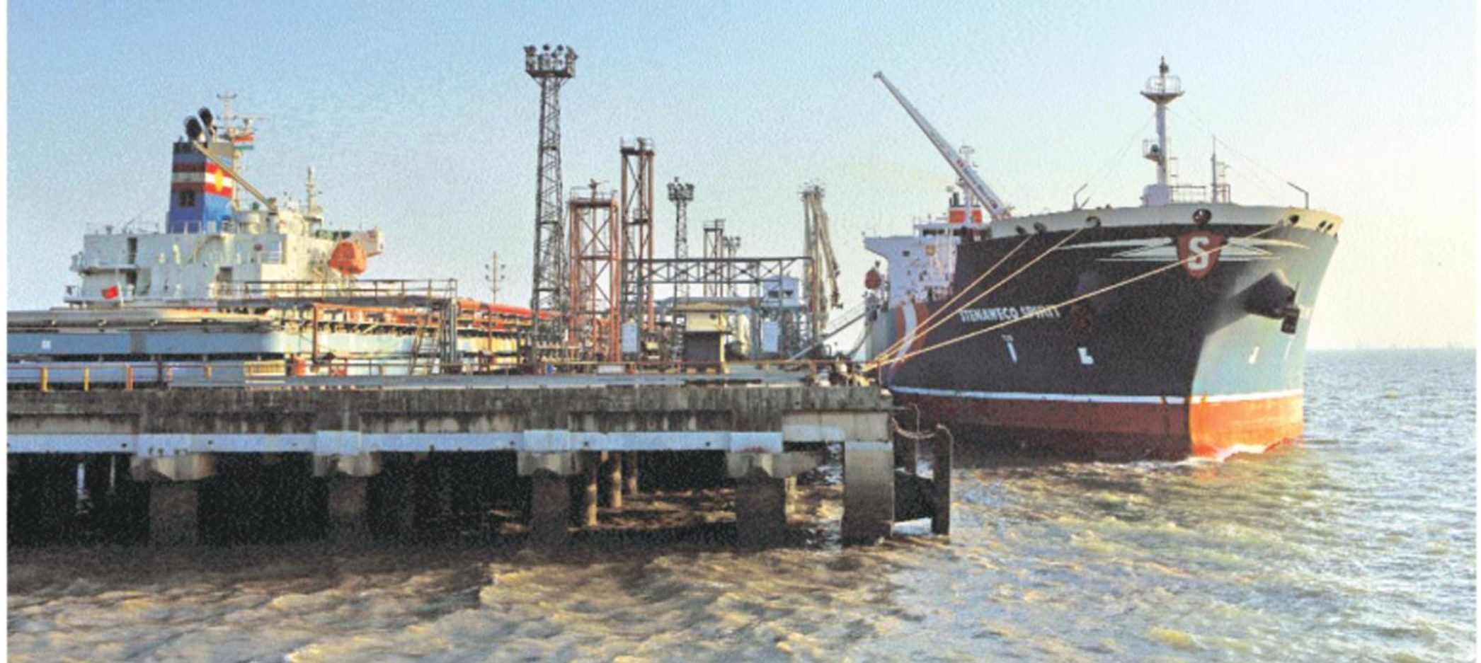
1. A SHIP IS ANCHORED AT THE LIQUID CARGO TERMINAL JOINTLY OPERATED BY BHARAT PETROLEUM AND INDIAN OIL CORPORATION
