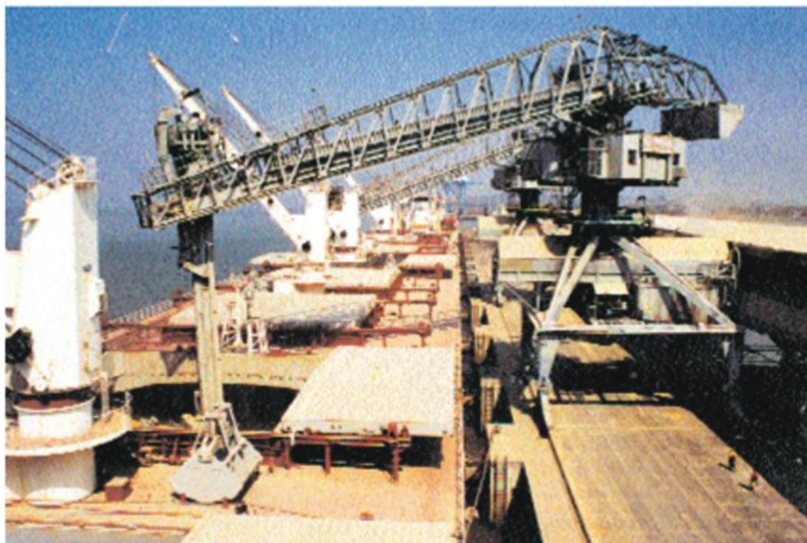
1. CONTINUOUS UNLOADERS INSTALLED AT THE BULK TERMINAL FOR BULK CARGO HANDLING. THE BULK TERMINAL WAS LATER DEMOLISHED TO MAKE WAY FOR A NEW CONTAINER TERMINAL.
