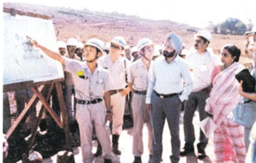
↑ (ABOVE AND BELOW LEFT) CIVIL ENGINEERS FROM JAPANESE CONSORTIUM MATSUI & CO. WITH JN PORT'S ANNA R. MALHOTRA AND BRIGADIER P.S. SETHI, PROJECT MANAGER (CIVIL)
