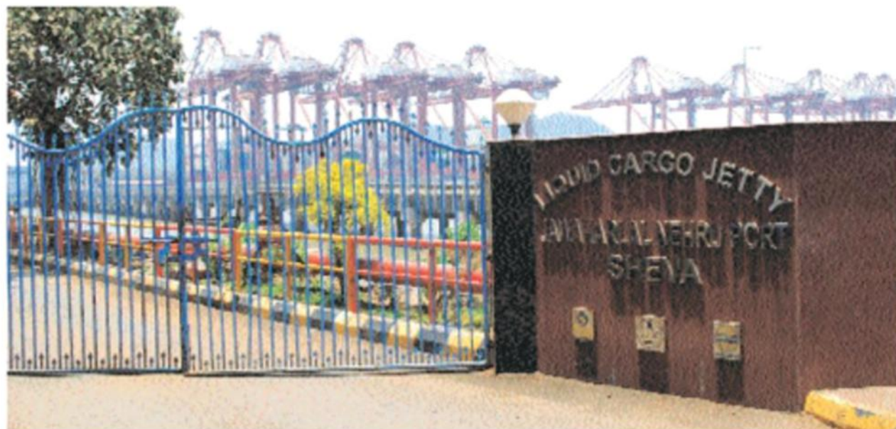
THE LIQUID CARGO TERMINAL AT JN PORT
