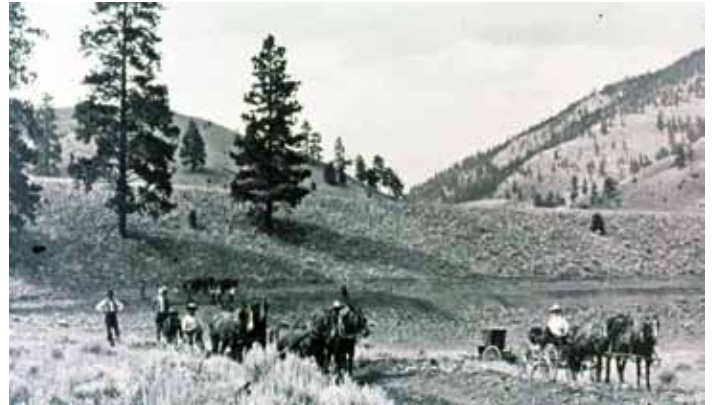
James Ritchie inspecting the irrigation works.
