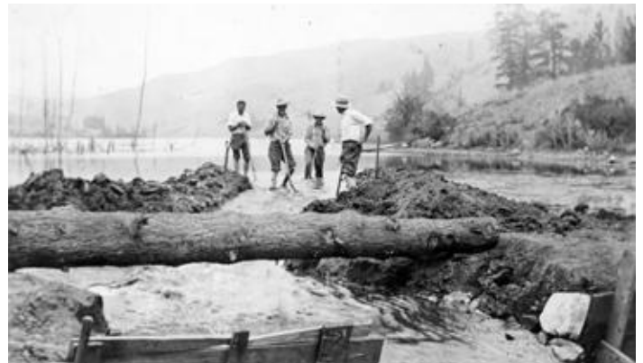
Brent Lake dam construction.
