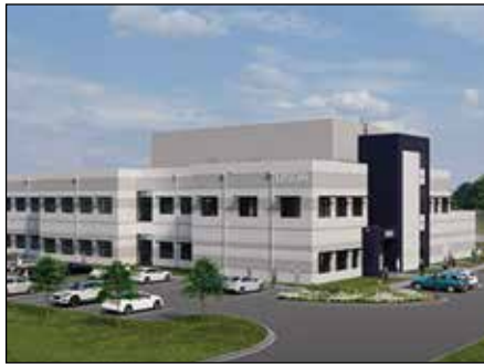
A rendering of the new Agricultural Research and Technology Center in Davis, California. (Image courtesy of Burns & McDonnell)
