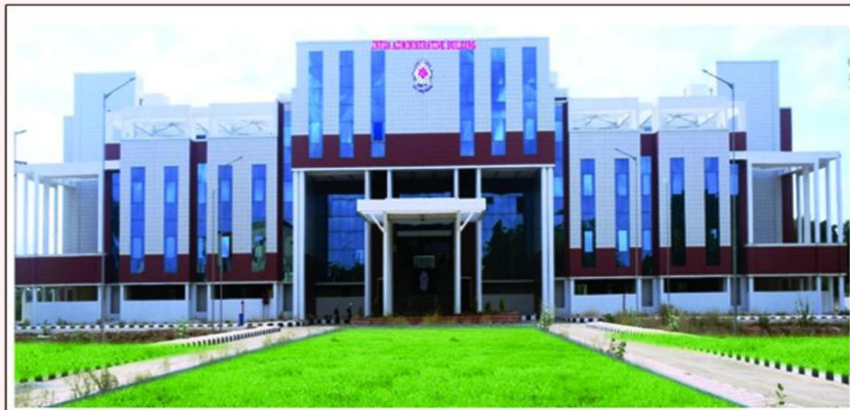
JNTUA ADMINISTRATIVE BUILDING
